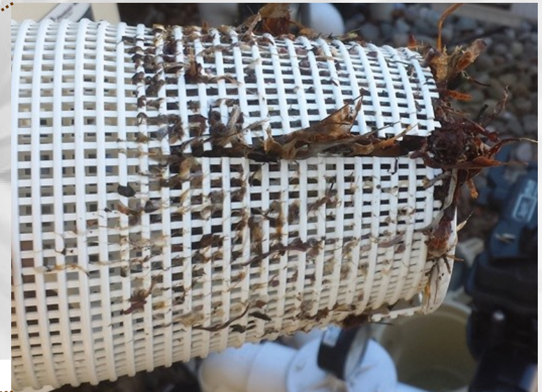
Fouled filtration system in a pump (source: internet)
